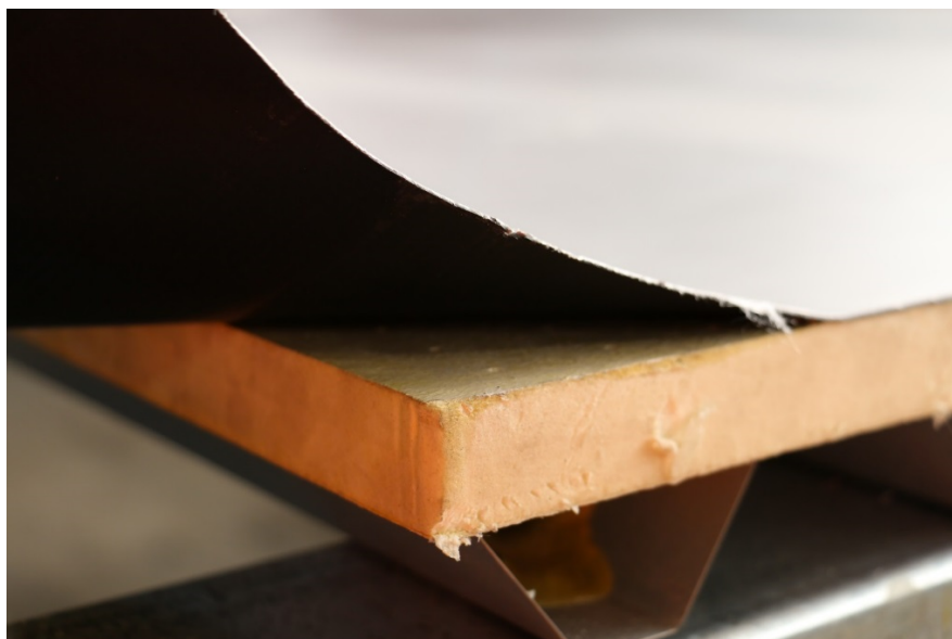
Figure 1: Cross-section of Warmspan Roof
