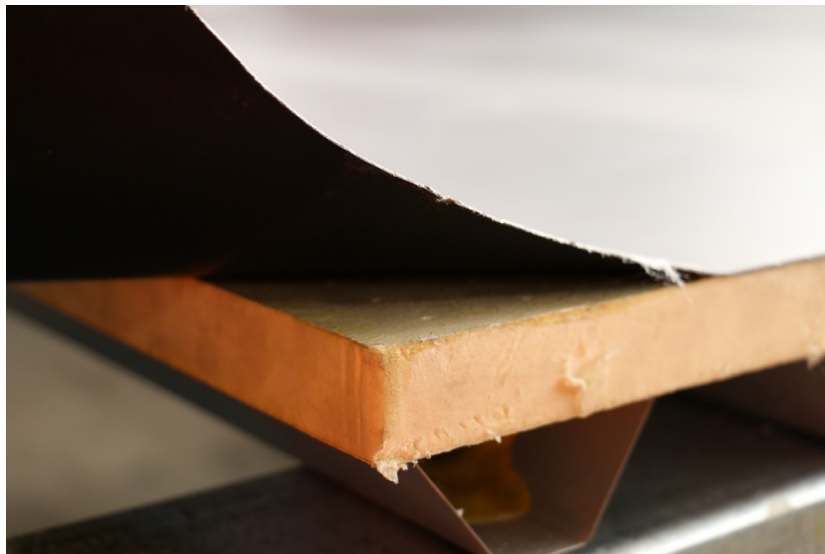
Figure 1: Cross-section of Warmspan Roof
