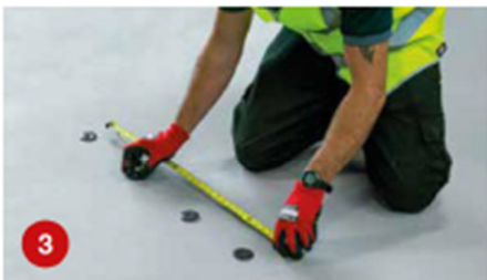
3. Apply fasteners for the application at centres determined by a Wind-Load Calculation.
