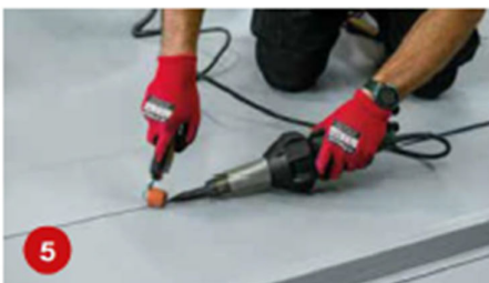
5. Hot-weld the 180mm wide membrane cover-strap to seal over the fixing line, taking pressure off the existing membrane.
