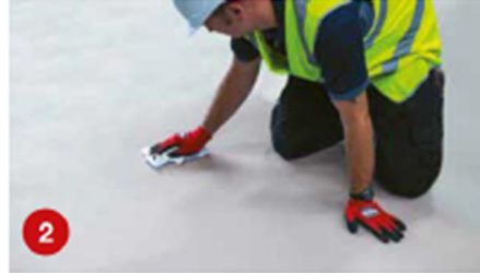
2. Clean surface with Viking Weathered Membrane Cleaner (STP001).
