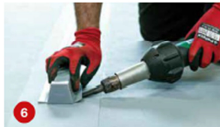
6. Hot-weld EJOBAR TPO 2G in the centre of the membrane, directly over the line of fasteners.
