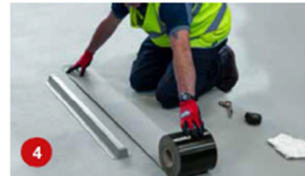
4. Prepare 180mm wide 1.52mm Enviroclad cover-strap rounding the ends, 100mm longer than the bar.
