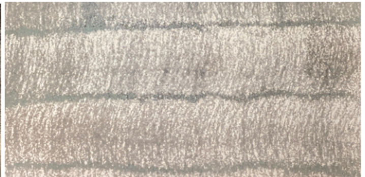
Proper Coverage on Insulation
