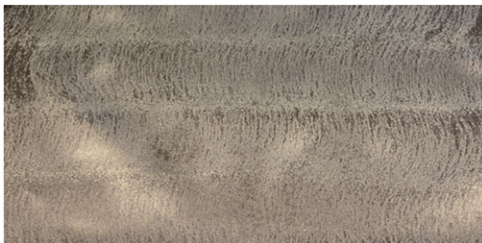
Proper Coverage on Membrane
